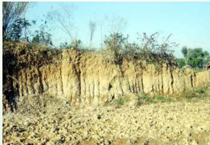
Plate.5. Waterlogging and salinisation are evident by moistened soil in the foreground and salt appearance on the field cuts
